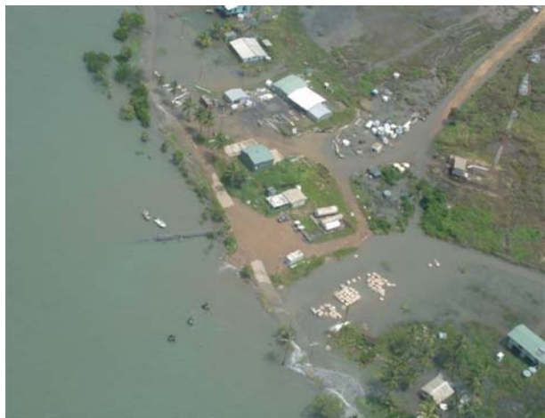
Fig. 5 Saibai village after inundation due to stormtides in 2006 (photo credit: Rick Parmenter)
